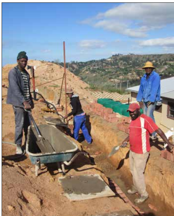
Digging the foundations
